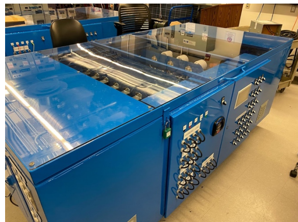
Figure 1: Benedum Power Lab bench from Eaton.
