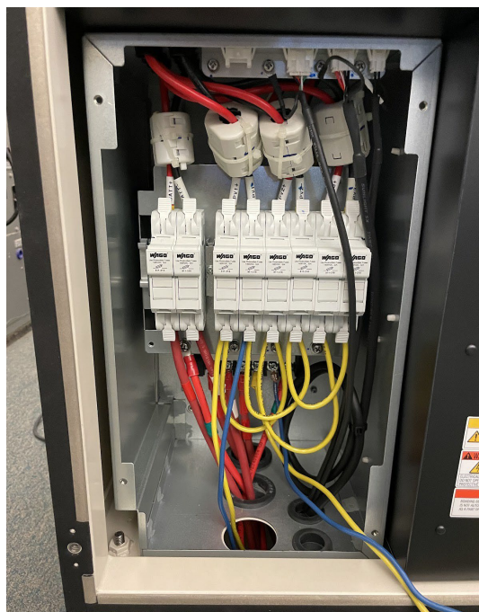
Figure 25: TabuchiInverter's Inputs/Outputs
